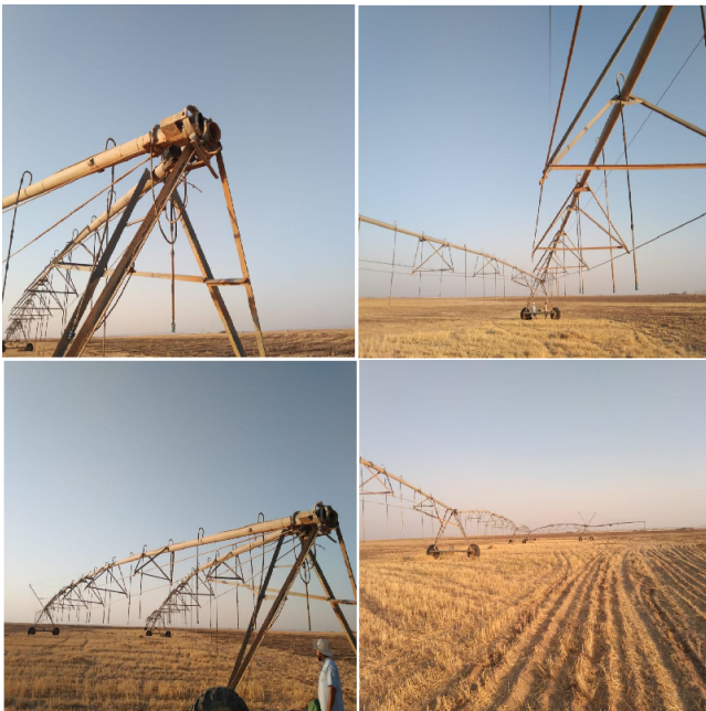
Fig. 1. Central Pivot Irrigation with damage.
